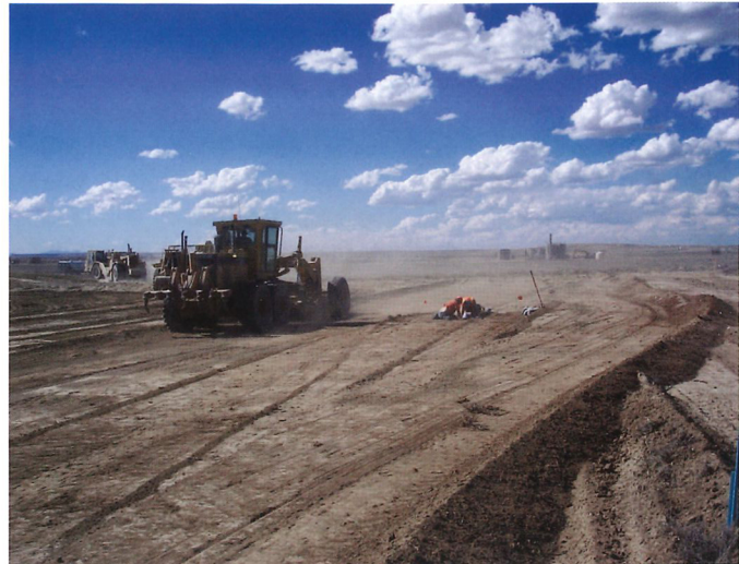
Archaeologists salvaging a feature discovered during construction in the Jonah Field. This is an excellent example of cooperation between the energy companies and the U.S. Bureau of Land Management.
