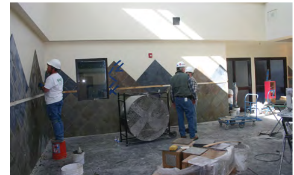
Workers continue finishing the interior of the elementary school in February, 2010.
