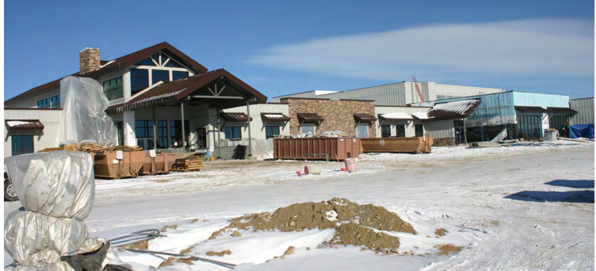
The new elementary school was closed in and heated in early November, 2009.
