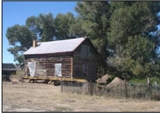
Sommers homestead house being prepped for its move to a new foundation.
