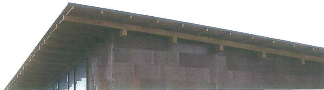
EXPOSED WOOD FRAMING
