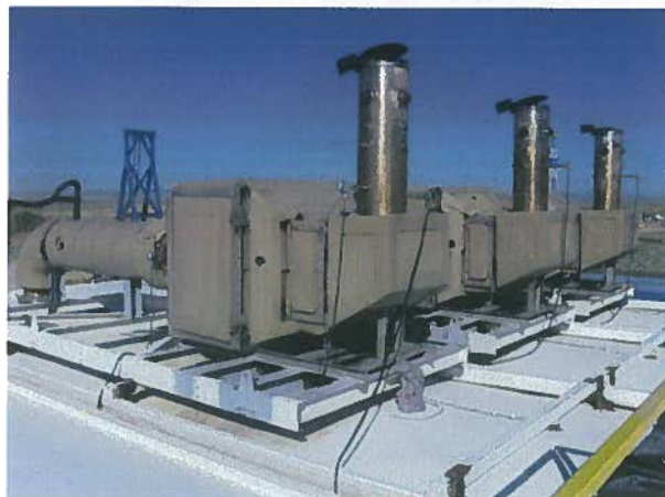
Figure 2. Three JM urea SCR systems installed above the engines
