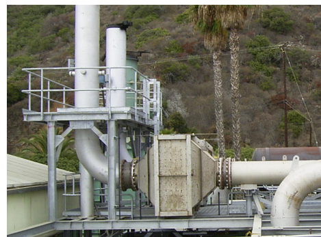
An installed SCR system.
